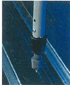
2. Drill Deck Holes
